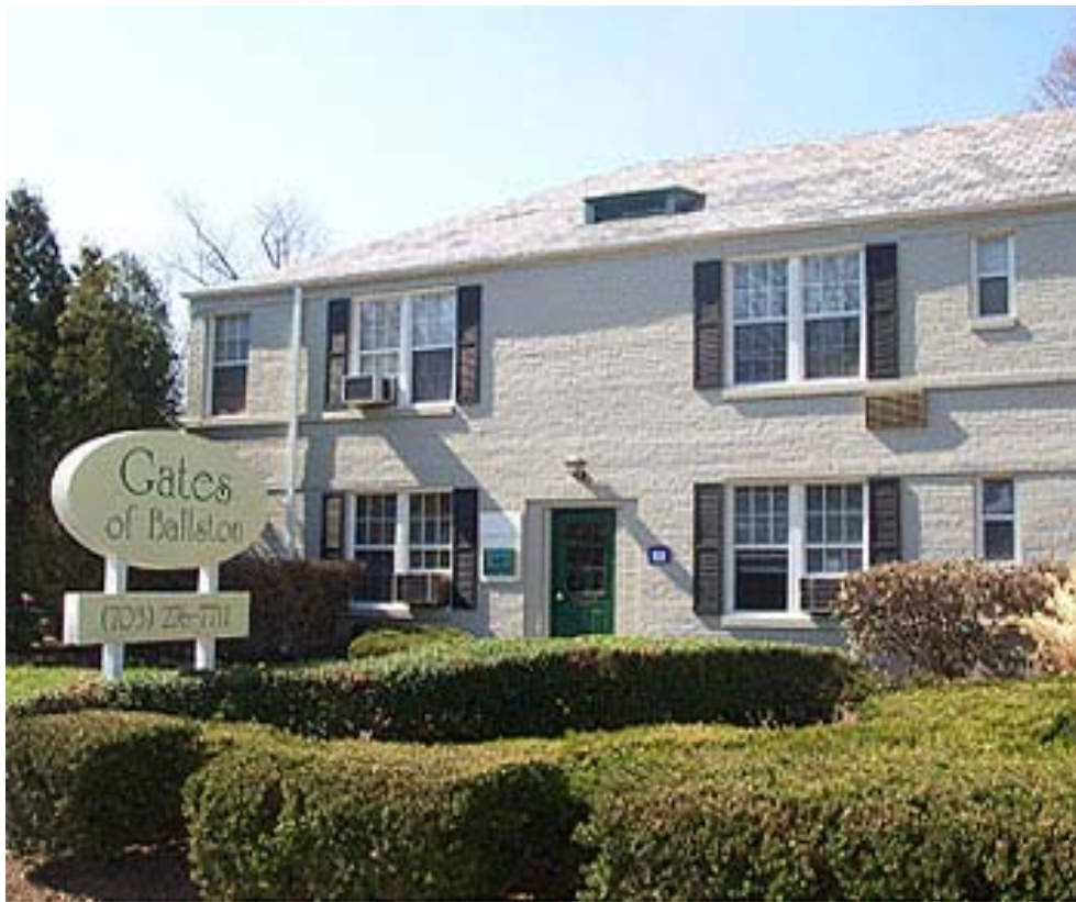
Gates of Ballston, 4207 Pershing Drive, Arlington, Va.
