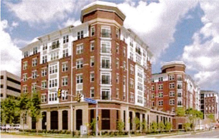
Avenir Place at the Dunn Loring-Merrifield Metro
